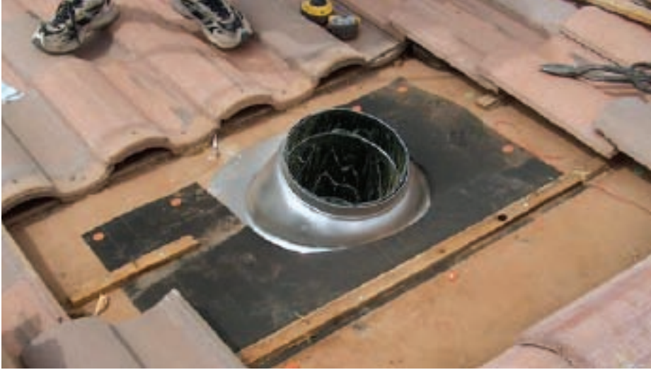
Photos courtesy of James Brown Roofing
