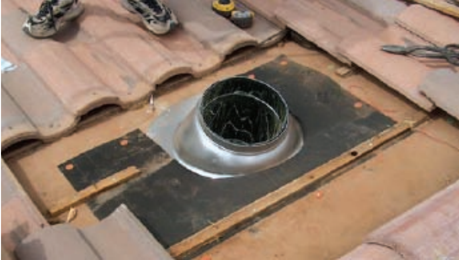
Photos courtesy of James Brown Roofing
